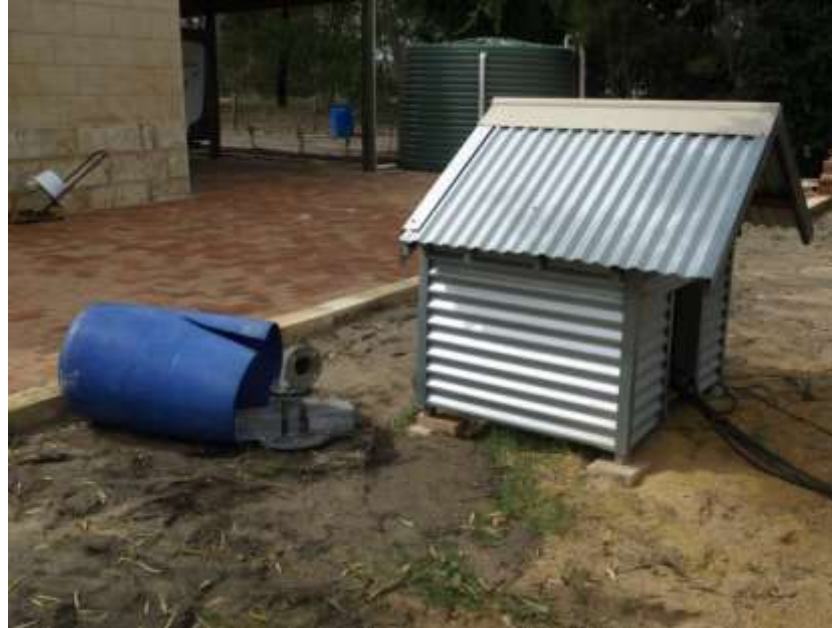
4. Bore and pump near workshop shed provides groundwater for lake input.
