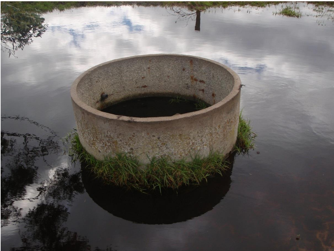
Plate 3. Soakwell present on site.
