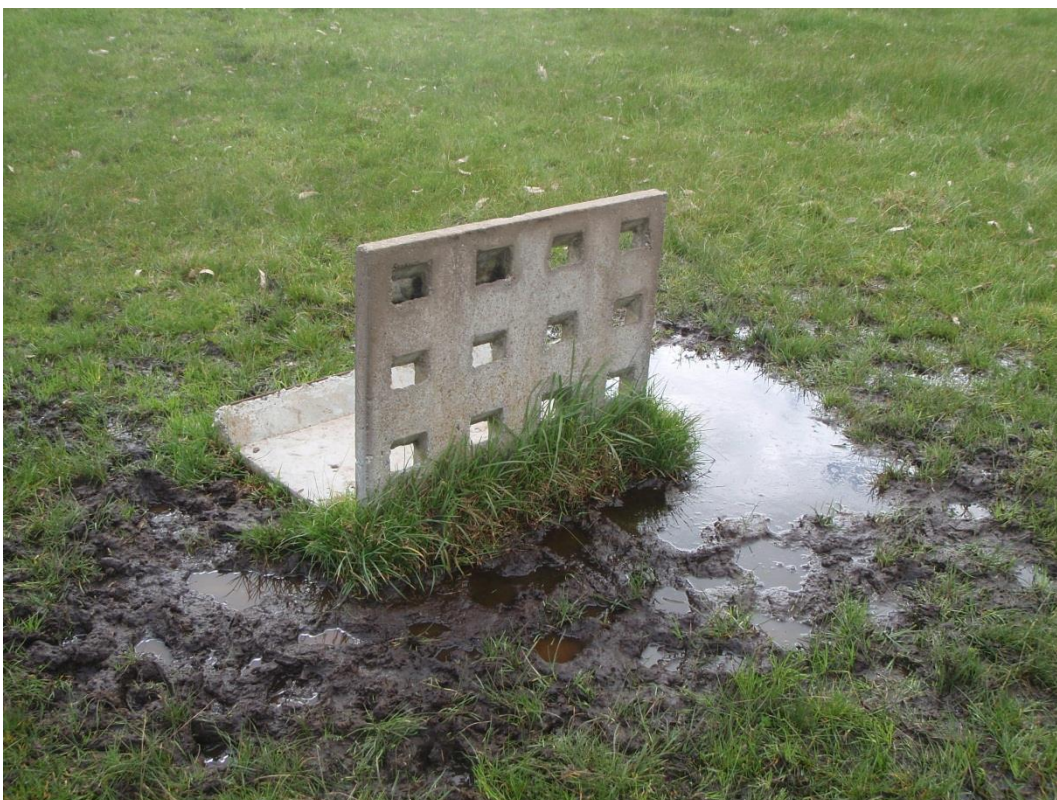
Plate 4. Soakwell present on site.
