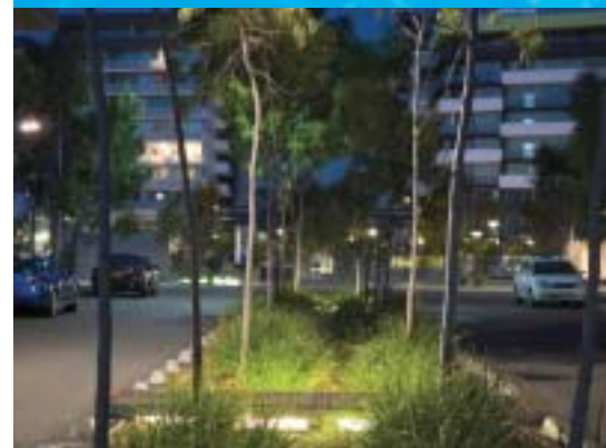
Victoria Park, Sydney – biofilter installation
