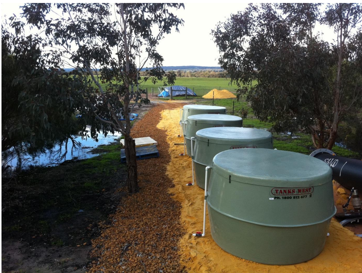
Figure 6: Photograph of Passive Treatment System prior to installation of inlet pipes
