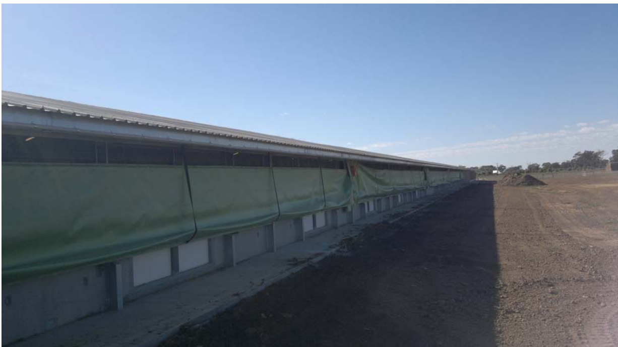
Exterior of Shed with Natural Ventilation Curtains opened 50%
