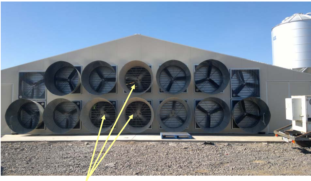
3 Fans Operating out of 14 Fans in total
