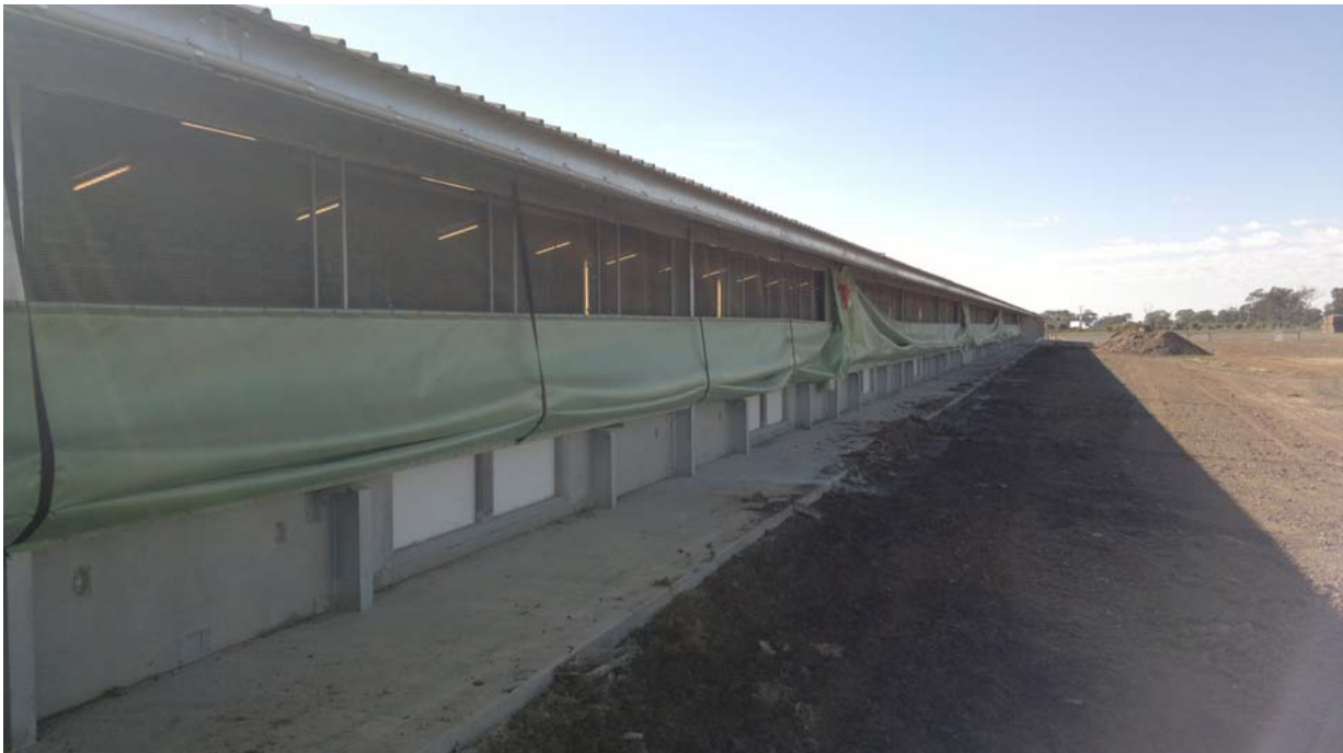
Exterior of Shed with Natural Ventilation Curtains fully opened
