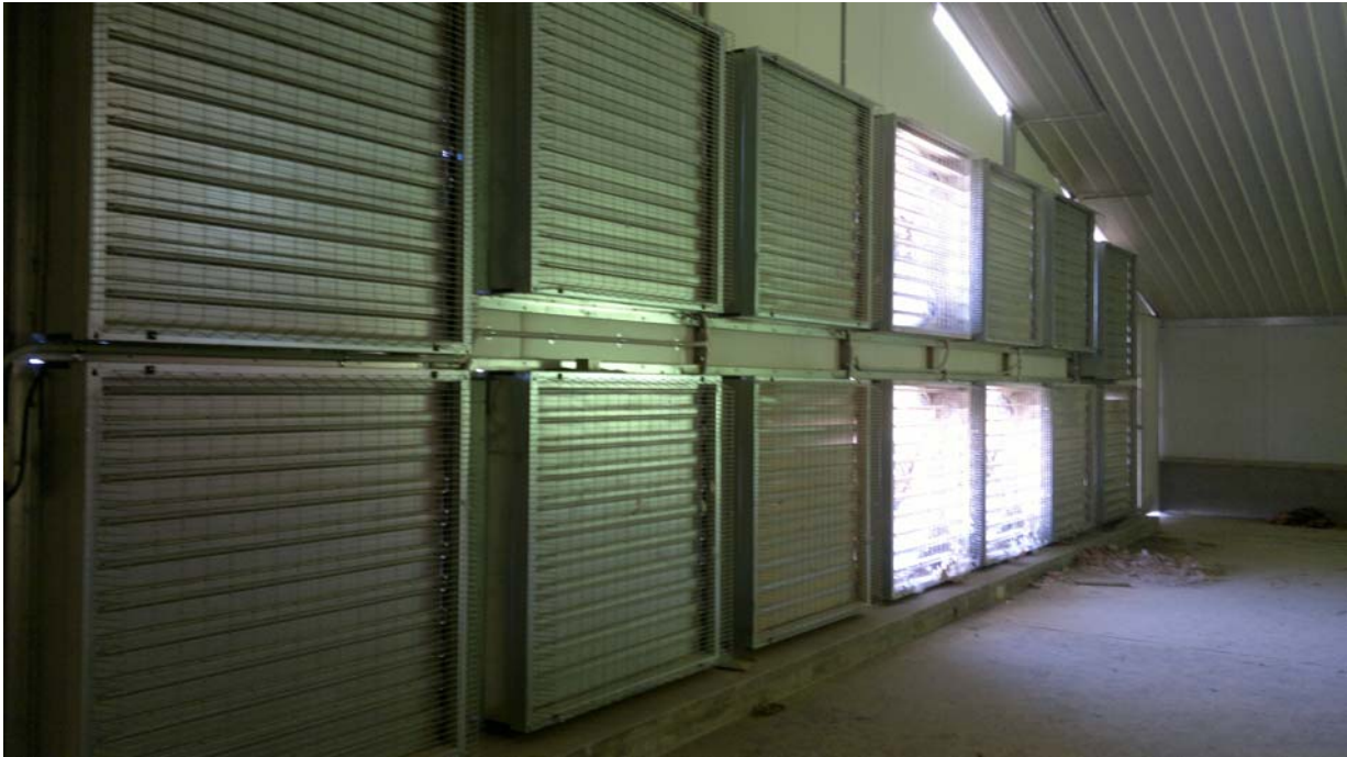
Interior of Shed showing back of Fans
