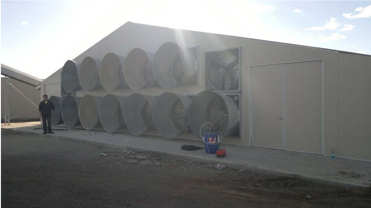
Rear of Sheds showing 14 x Fan Configuration
