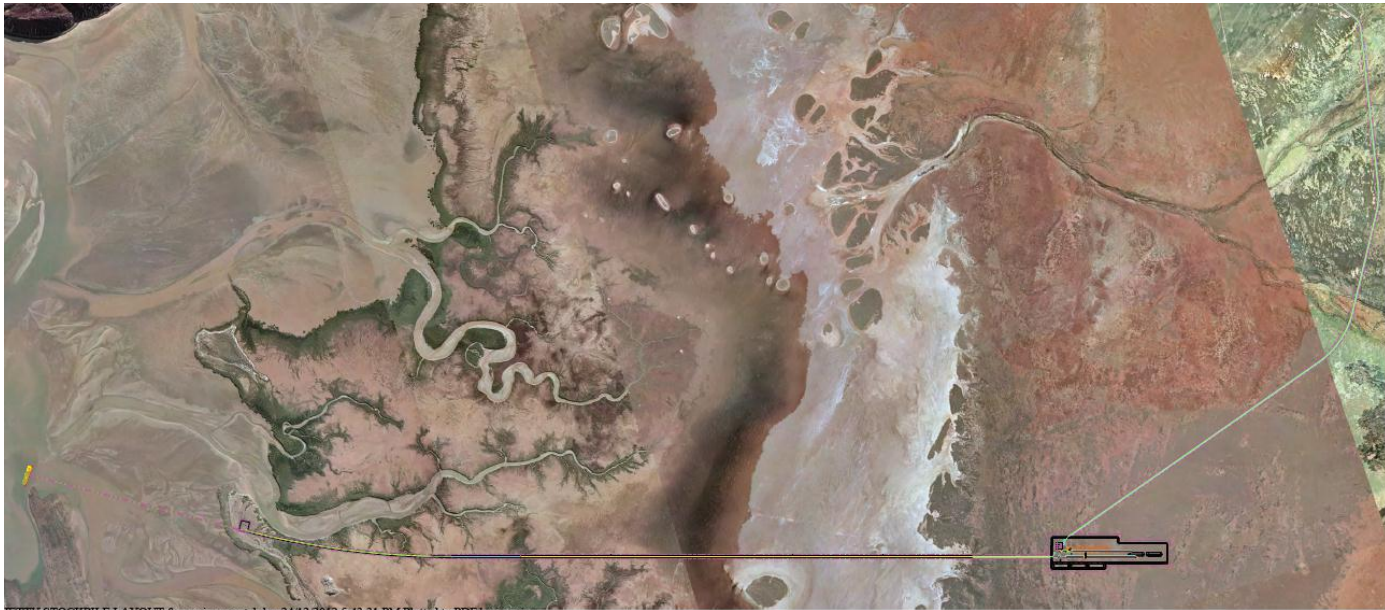
Figure 2 Proposed slurry pipeline to the iron storage area and the conveyor route to the ship loading facility.
