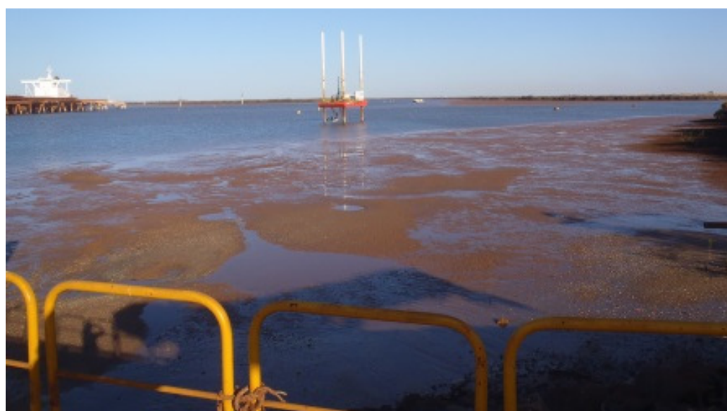
Figure 2-3: Tug Haven site facing east from Australia Island, with AP3 on the left.
