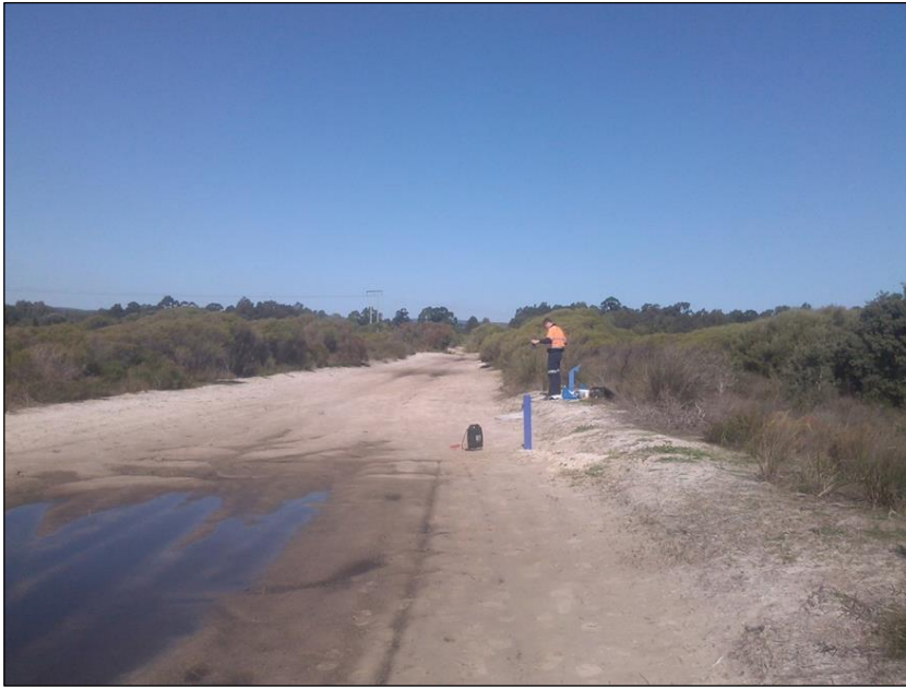
Figure 3: Existing fire access track on pipeline alignment (facing southeast)
