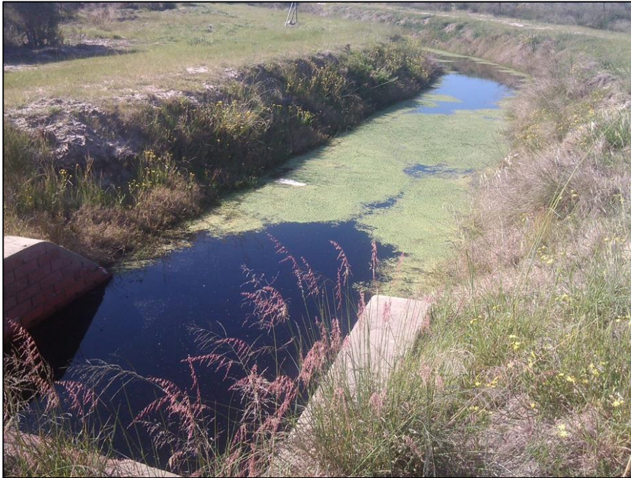
Figure 20: Baileys Branch Drain with levee banks
