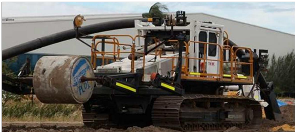
Figure 2: EcoPlough installing a PE pipeline
