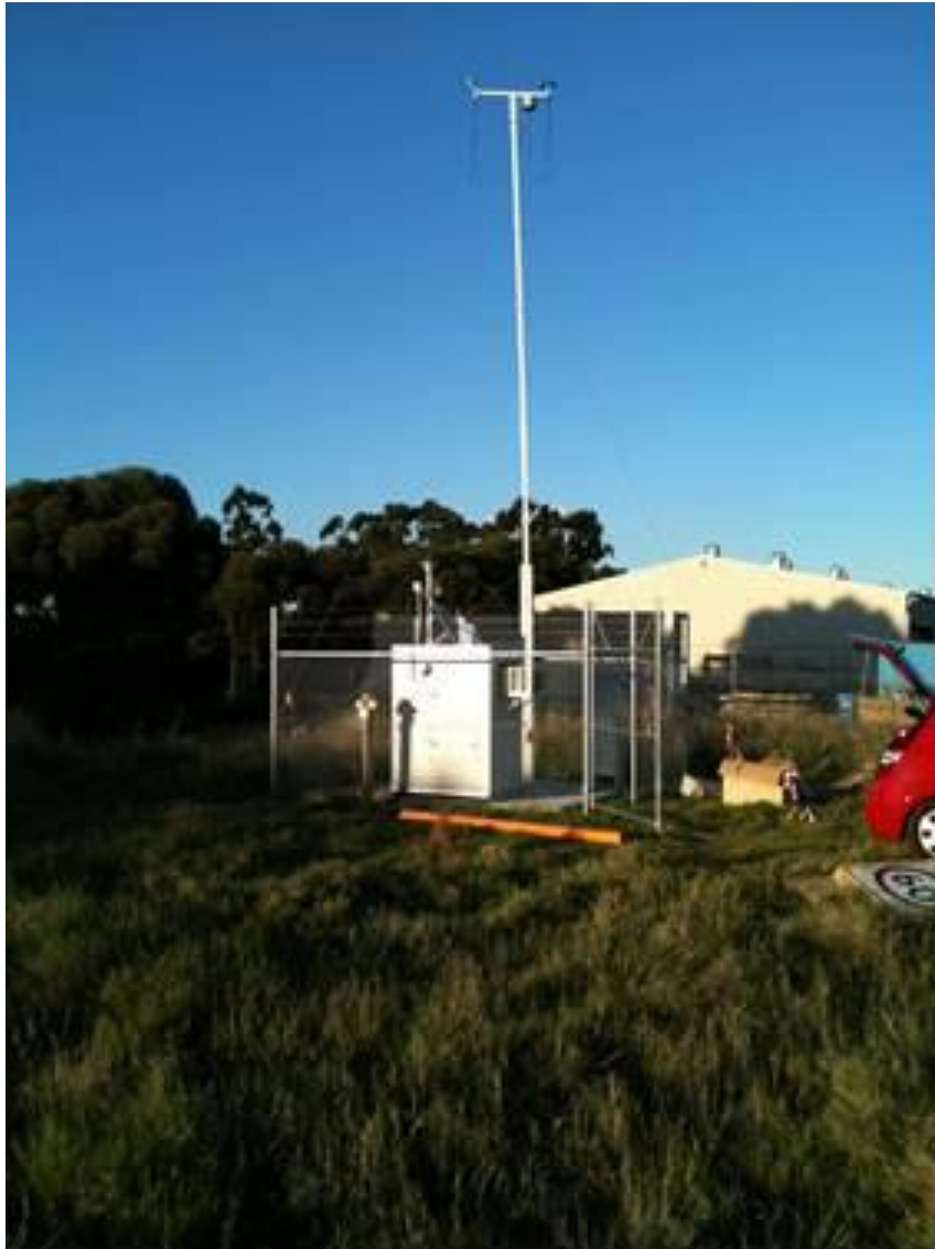
WA Limestone AQMS – Weather Station, TEOM & HVAS
