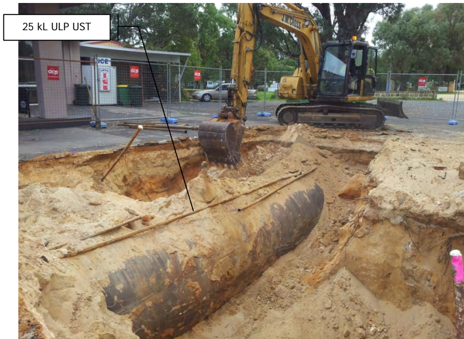
Exposing 25 kL ULP UST – view to the north north-west
