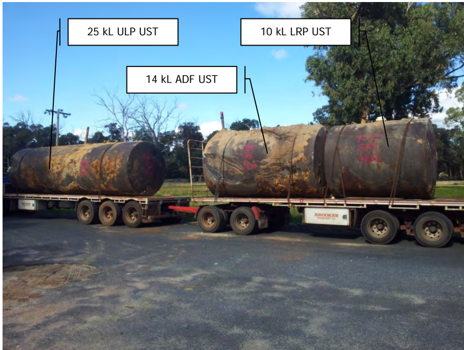
All three USTs secured for transport
