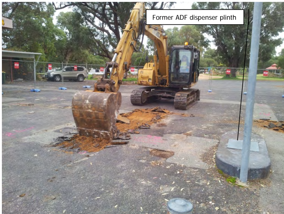
Starting surface removal and excavation works – view to the north-west
