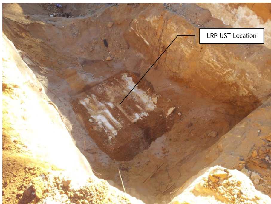
Limestone base below 10 kL LRP UST location – view to the north-east
