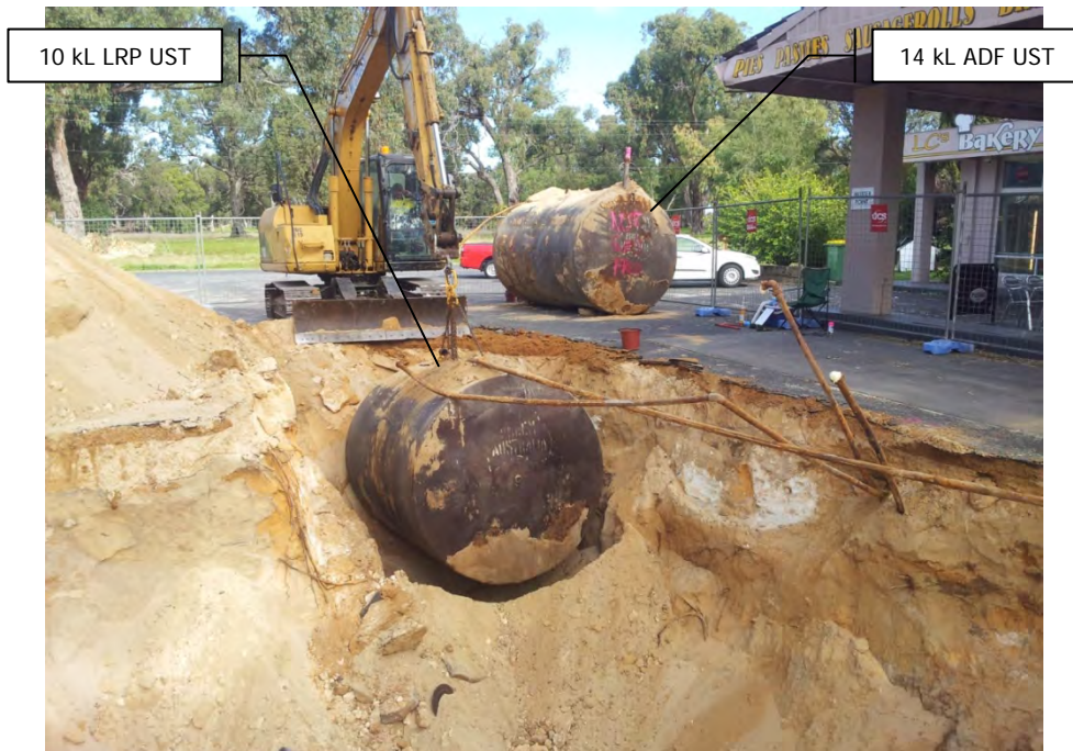
Removing 10 kL LRP UST– view to the south south-west
