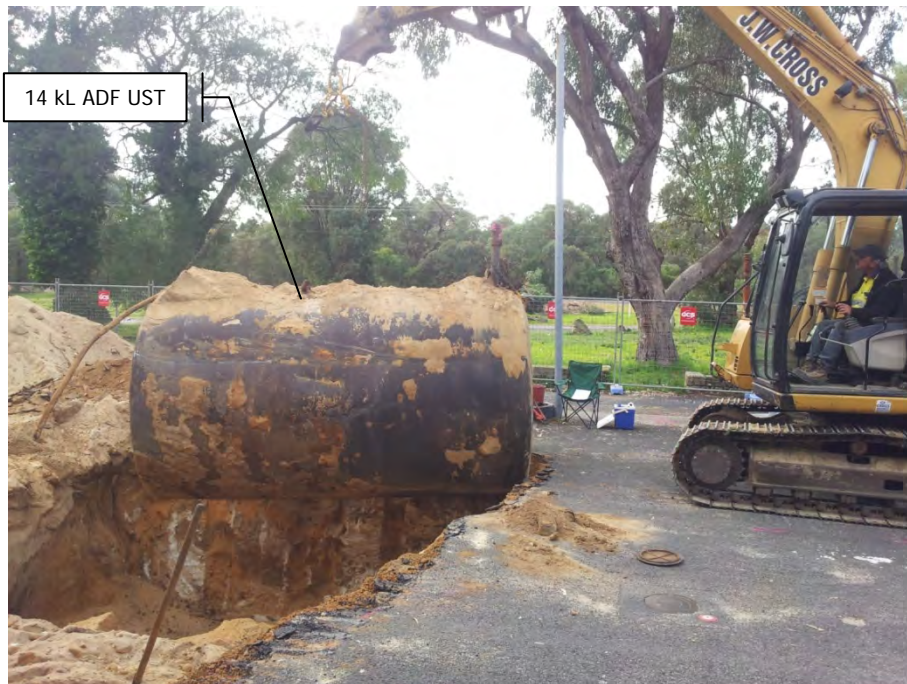
Removing 14 kL ADF UST from ground – view to the east, north-east
