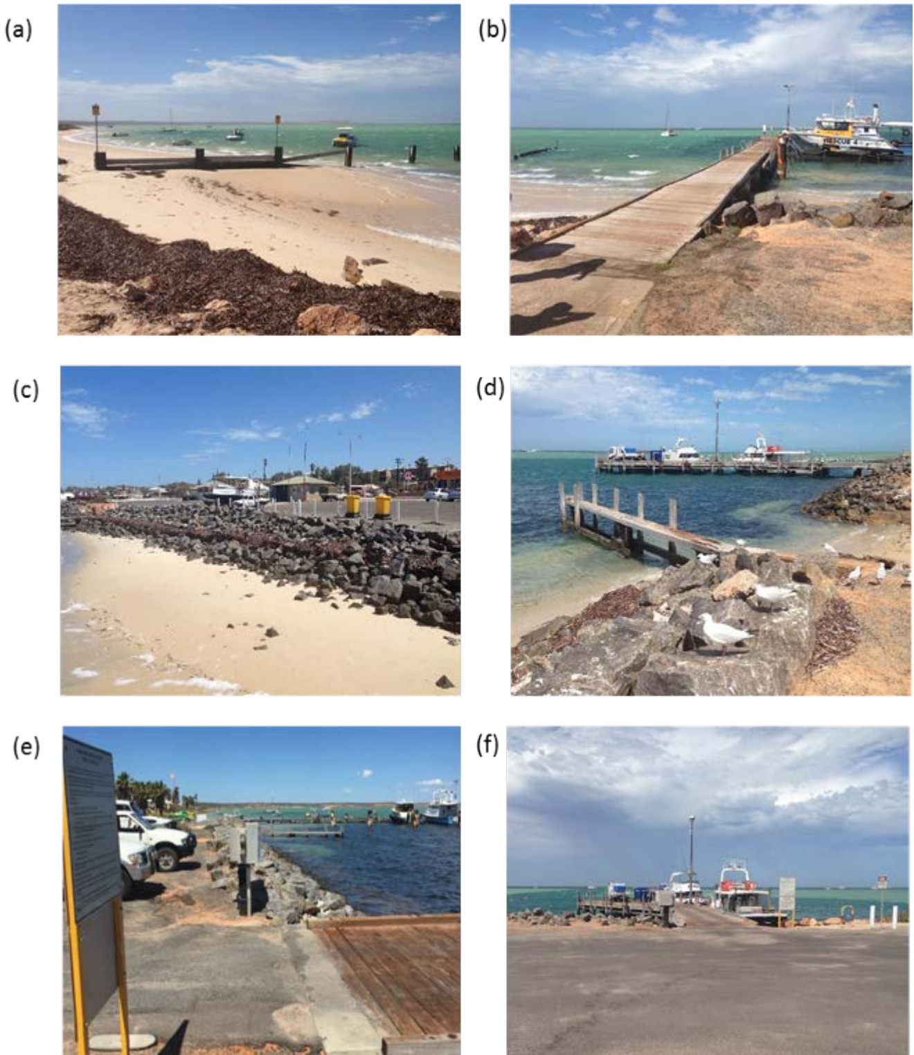
Figure 3-2 Site photographs showing shoreline features: a) timber groyne and beach to the southeast of the project area; b) recreational jetty; c) rock revetment between the recreational jetty and the jinker ramp; d) timber finger jetty and seaward edge of slipway/jinker ramp; e) rock revetment between the service wharf and slipway/jinker ramp; and f) service wharf.
