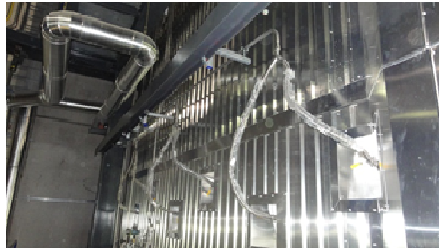
Figure 18: View of SNCR injection lances
