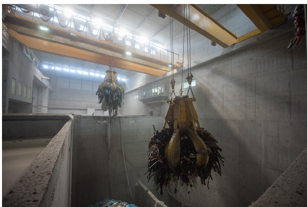
Figure 9: Photo of overhead crane in a WtE plant
