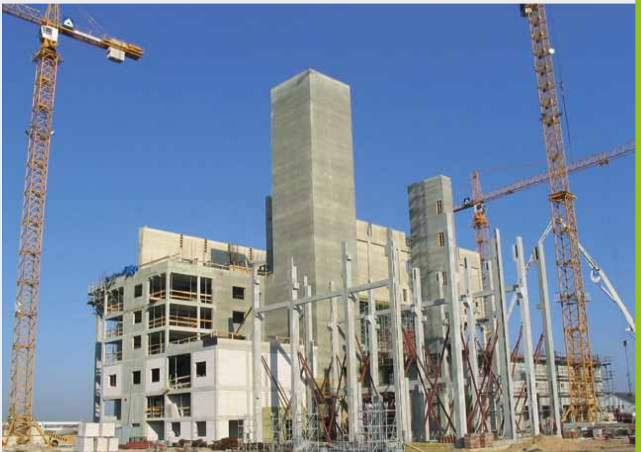
EfW plant under construction in Zorbau (Germany)
