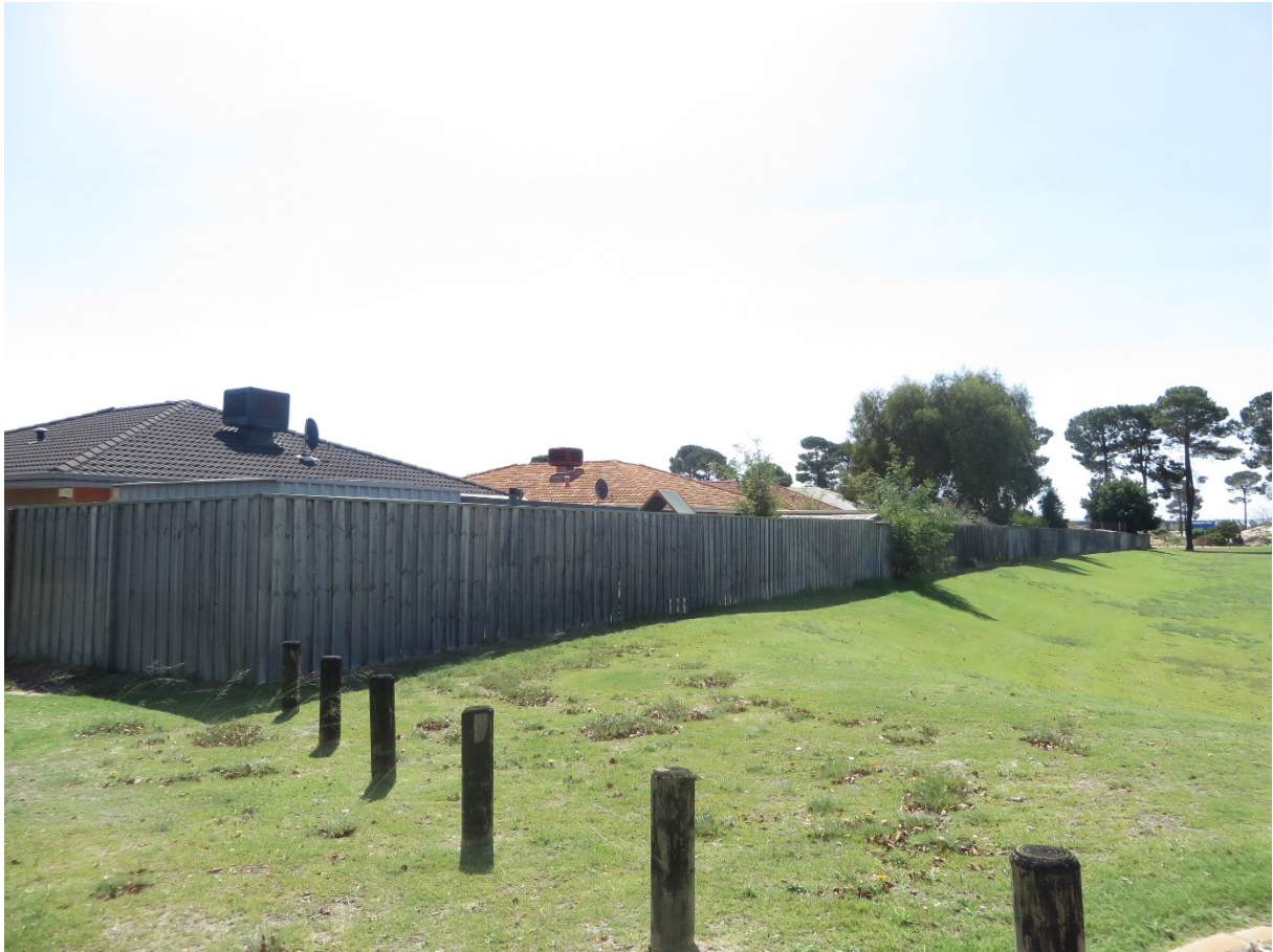
Feature walls could offset noise impacts and balance perceptions of loss of land value should they replace timber fencing such as for these dwellings fronting Vaucluse Crescent, Ellenbrook.
