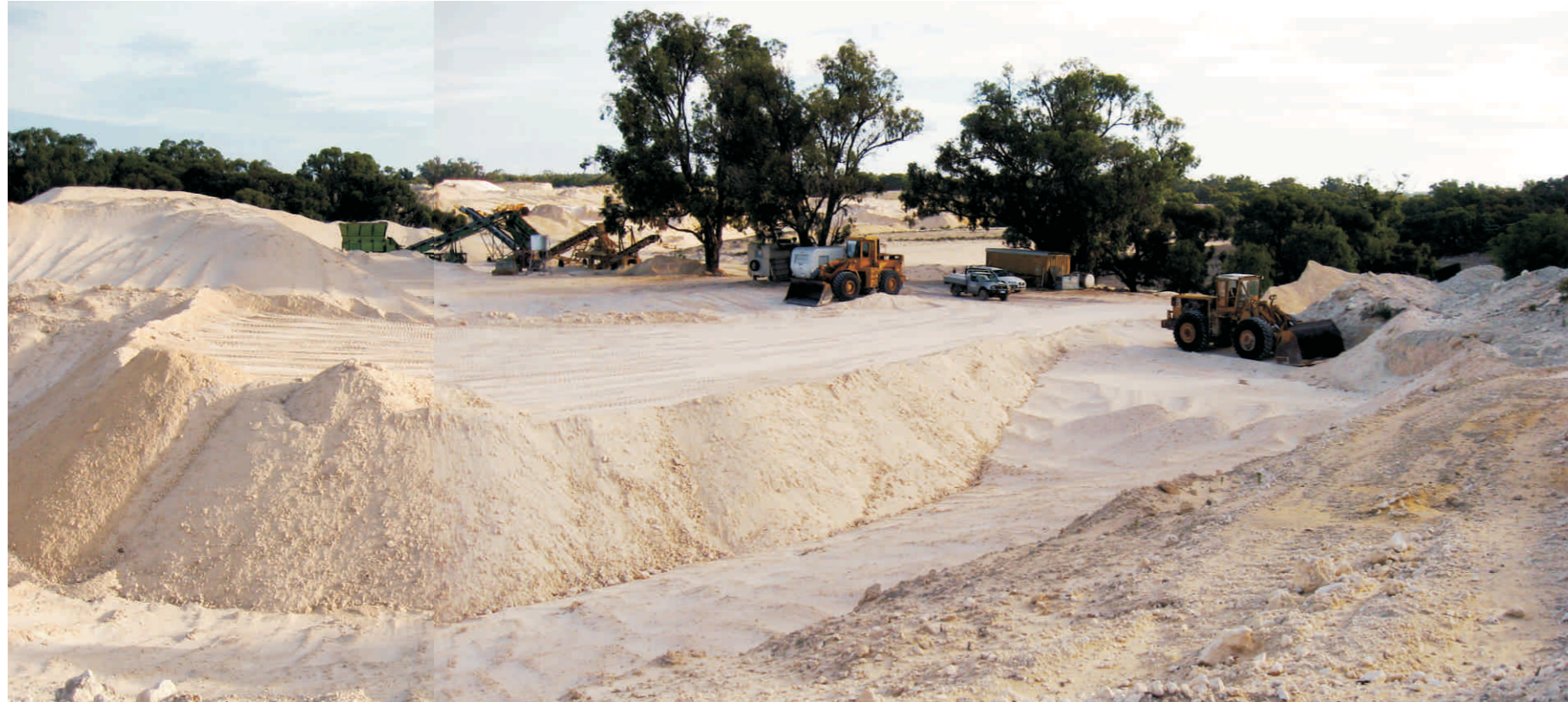
Doyles Lime typical operations at Myalup pit. Operations will be similar at the proposed Preston pit.
