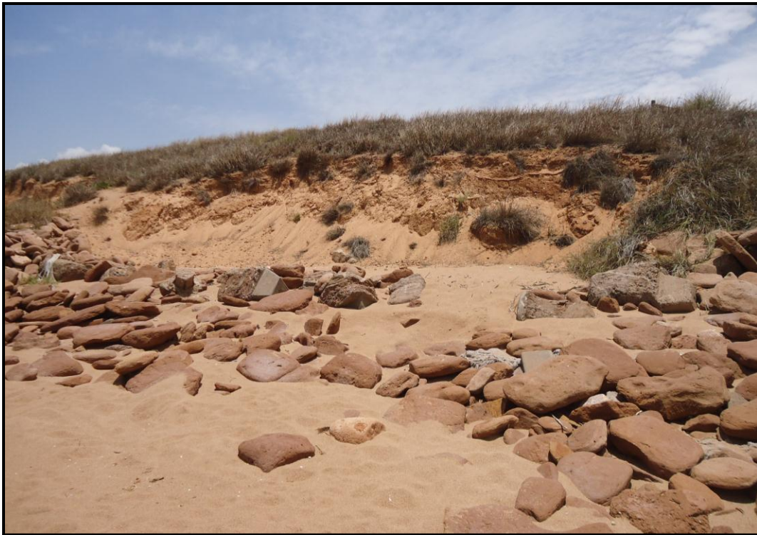
Plate 17: The beach below Sutherland Street, Port Hedland, showing the erosion that occurs during storm surges. The retaining embankment has been torn down by wave action.
