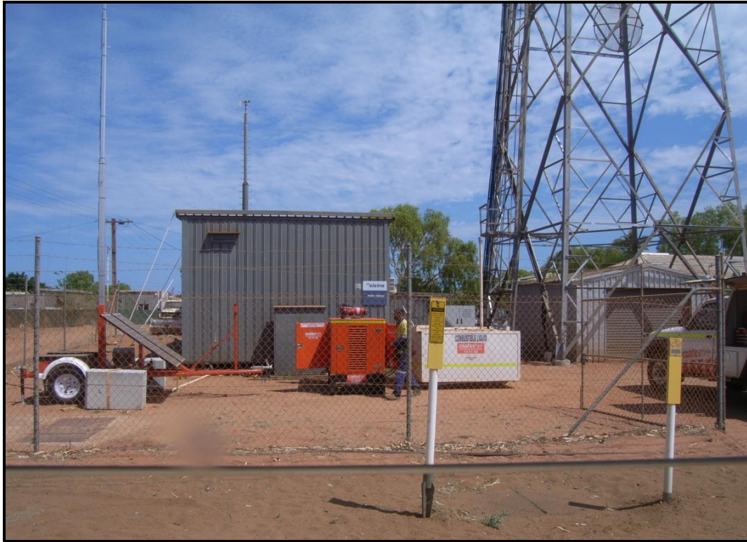
Plate 11: This possible site for the CEV building at Onslow was rejected by the Company as being already too crowded with Telstra equipment.
