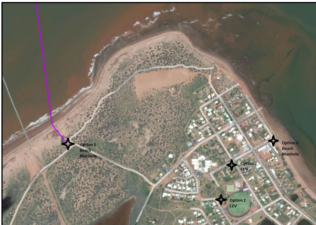
Figure 1: The proposed project development areas at Onslow. All four sites were inspected (image supplied by the Company).
