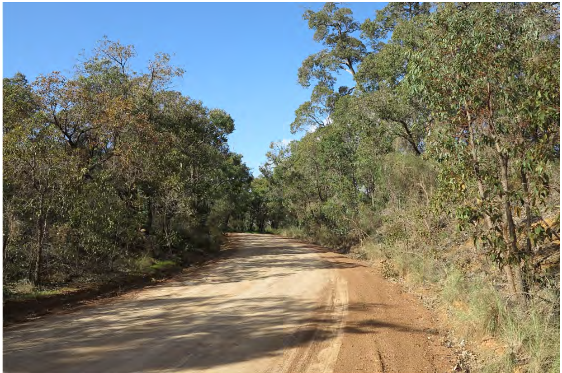
Figure 6 – 5 Section of Pruden Road near South western Highway that will require widening by about 2 metres
