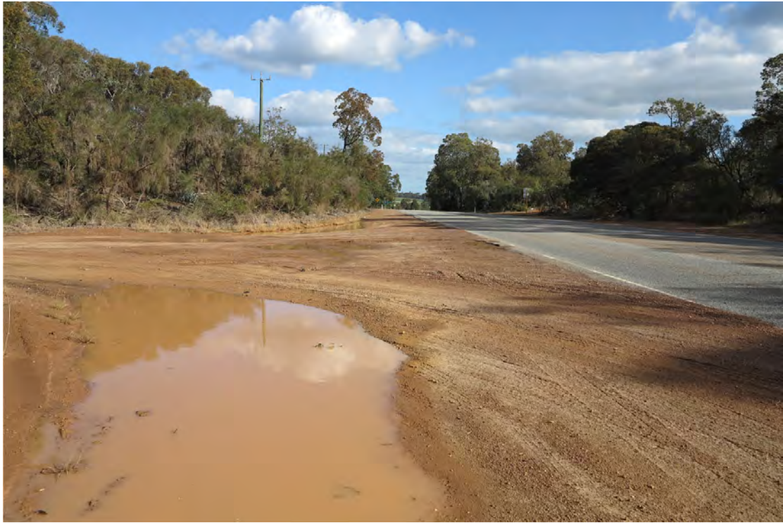
Figure 4 – 3 Pruden Road crossover to South Western Highway, view south
