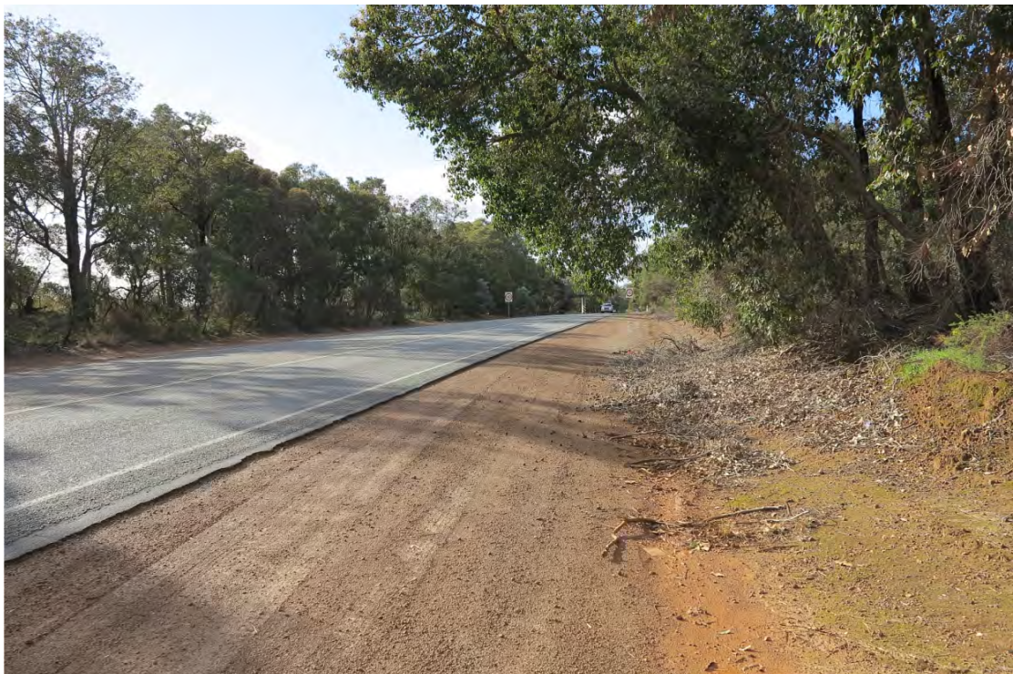
Figure 4 – 4 Pruden Road crossover to South Western Highway, view north
