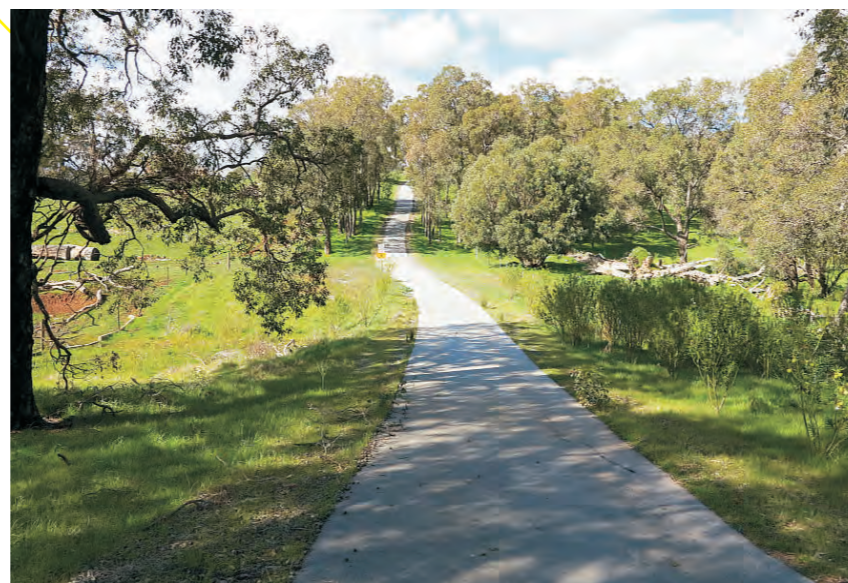
Pruden Road, view east
