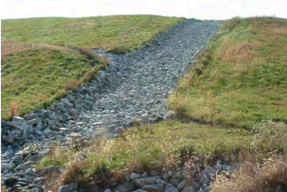
Figure 2 - 8 Examples of rip rap and stone pitching to manage water on slopes, slow the water flows. All detention basins will be provided with rock pitching to protect the outlets
