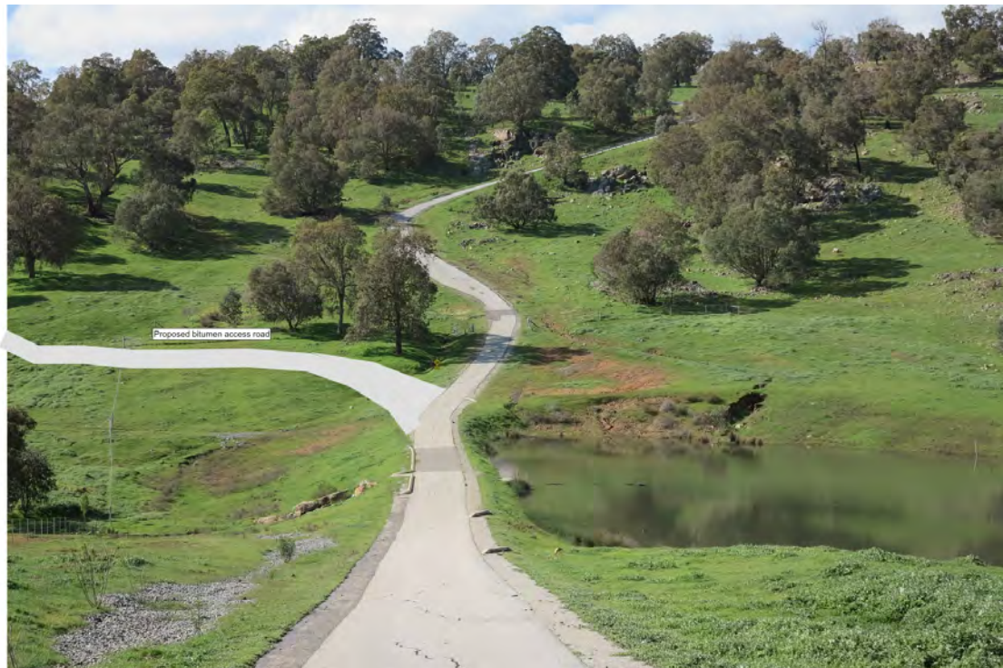
Figure 4 – 8 Existing access and proposed access road on Lot 800, view north.
