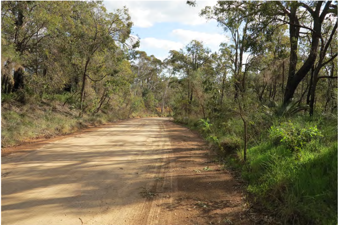
Figure 6 – 6 Section of Pruden Road near South western Highway that will require widening by about 2 metres
