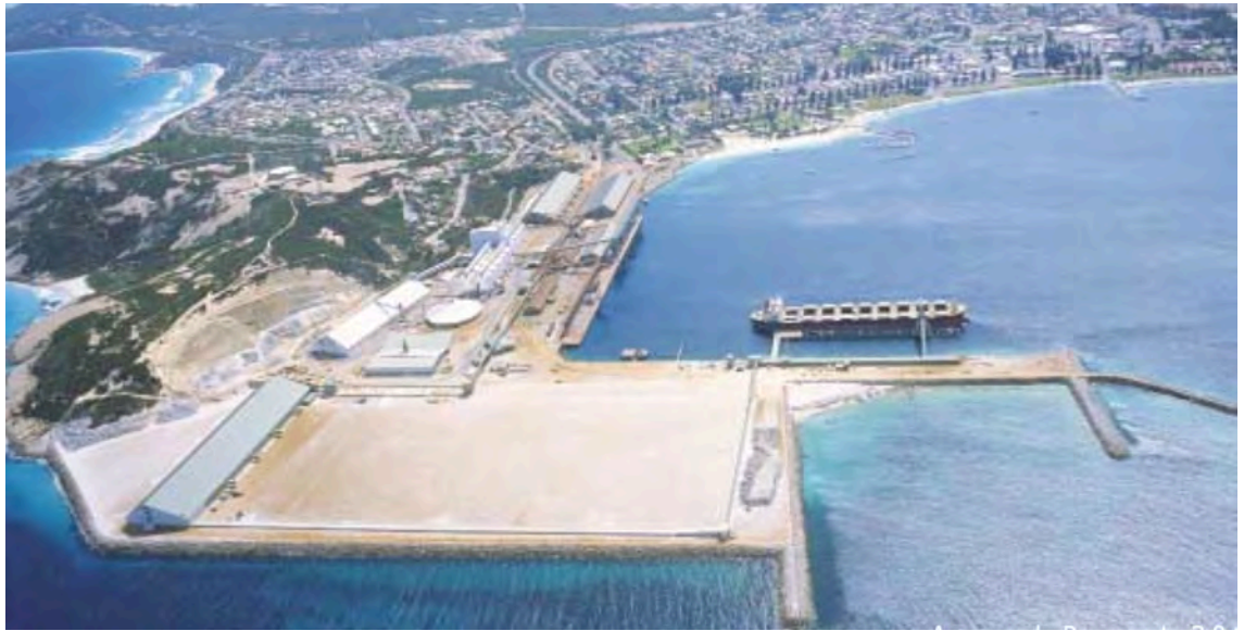
Figure 4 – 1 Esperance Port 2004 – Note the bare ground of the completed quarry to the left of the large sheds
