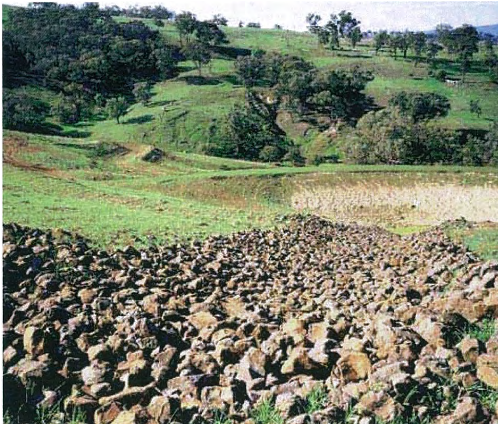
Figure 2 - 7 Examples of rip rap and stone pitching to manage water on slopes, slow the water flows. All detention basins will be provided with rock pitching to protect the outlets
