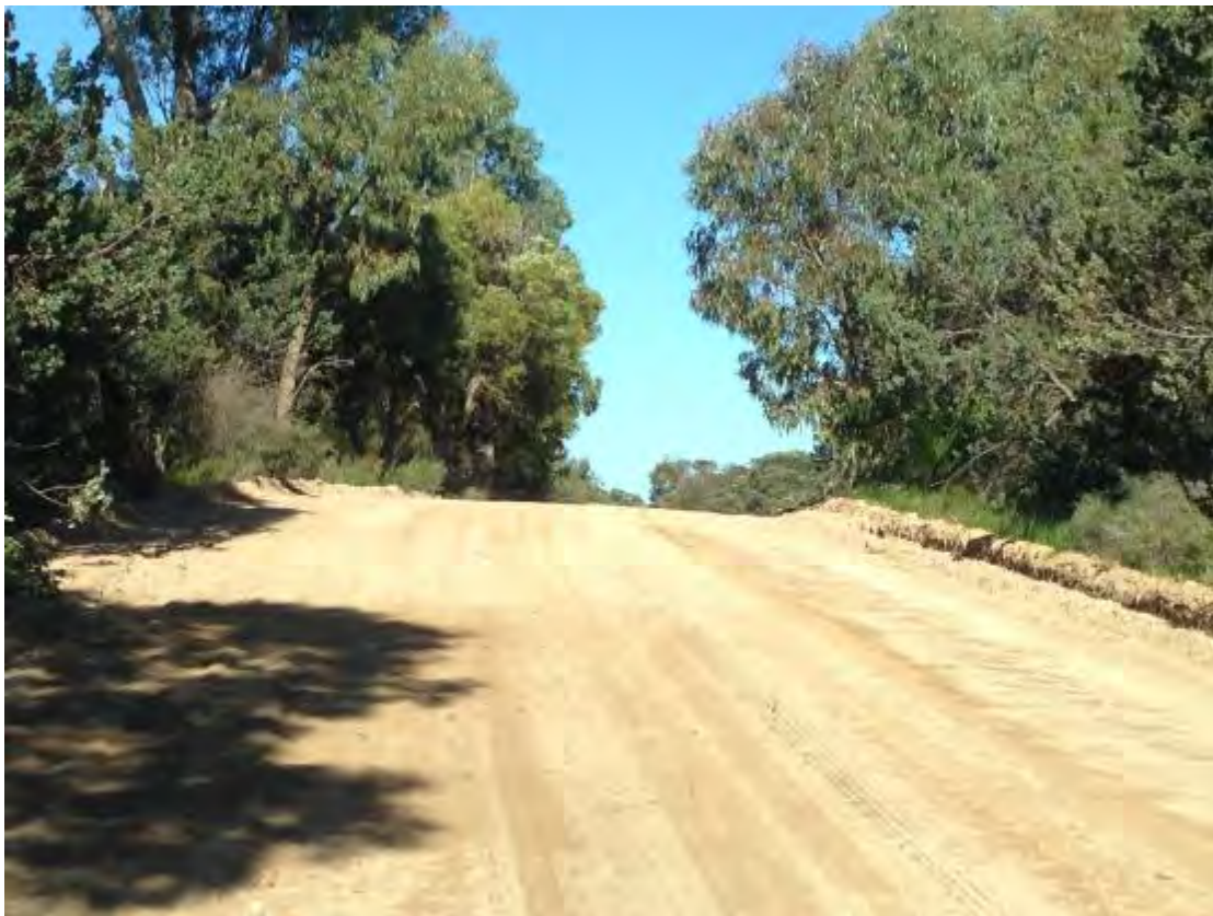
PBR North, SLK 4.3 blind crest on curve just south of campground turn-off.
