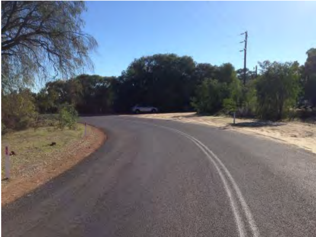
Preston Beach Road, approaching PBR North intersection. Intersection location determined by maximising sight distance on curve.
