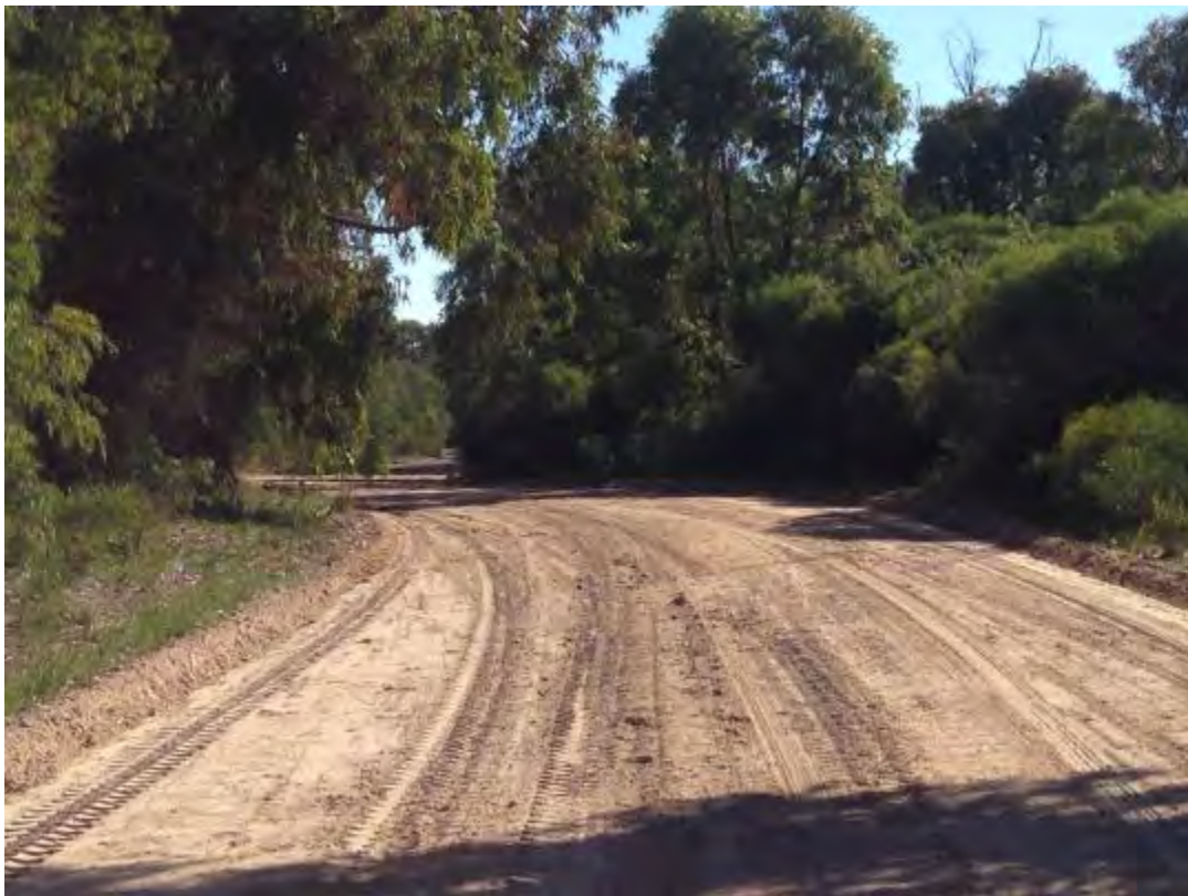
PBR North, SLK 1.4, typical 6.5m wide track, overhanging vegetation
