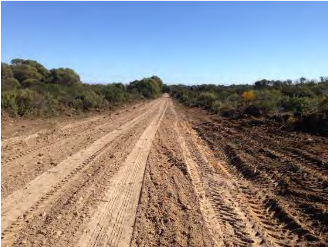
PBR North SLK 5.0, looking north
