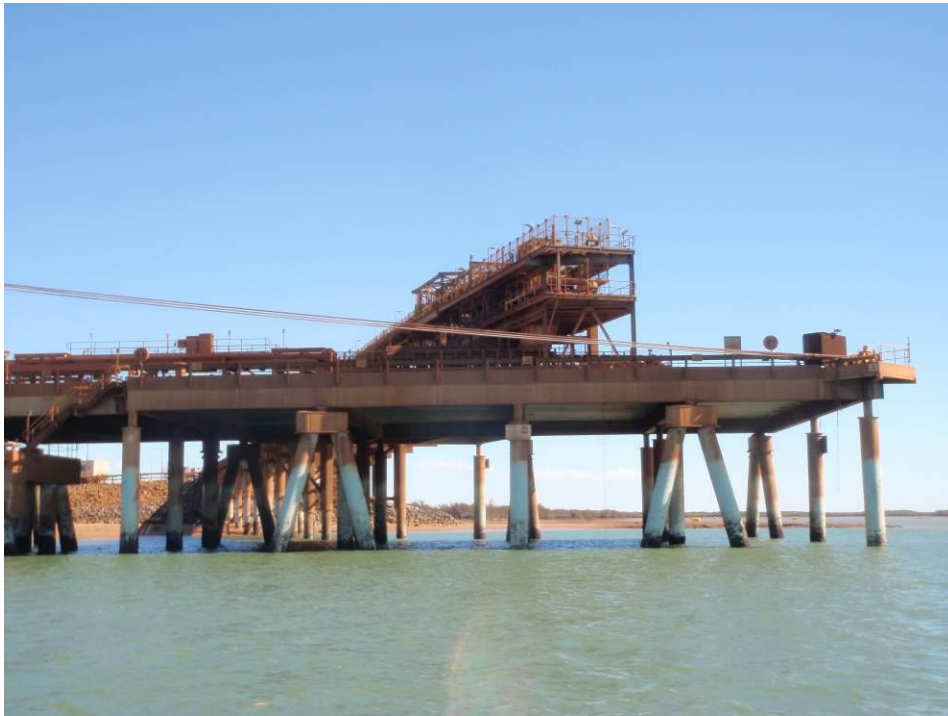
Figure 9: Similar piles and wharf structure
