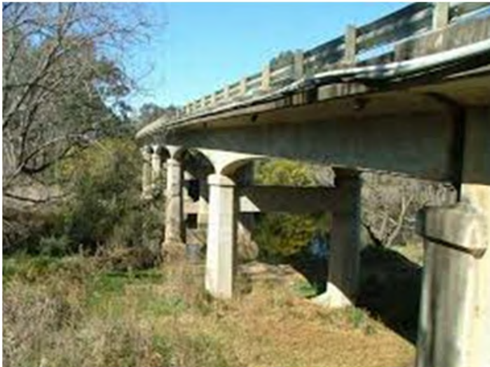
Plate 5 Bemboka bridge in NSW
