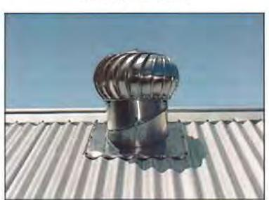
Figure 5: Typical Roof Ventilation
