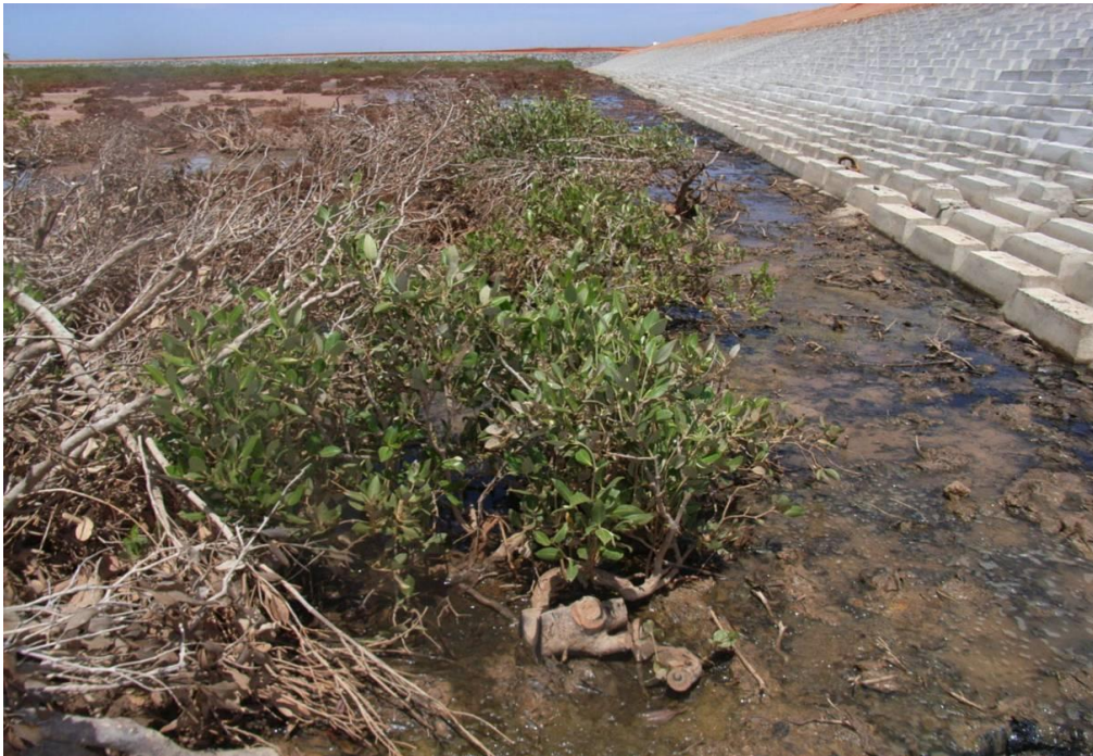
Plate 2 Vegetative recovery of cut Avicennia mangroves at the base of perimeter bund
