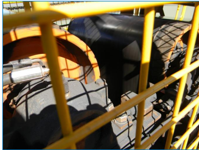
Figure 3-3: Fugitive emissions and build up of material around pulleys
