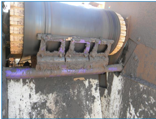
Figure 3-1: Scrappers on head end of conveyor
