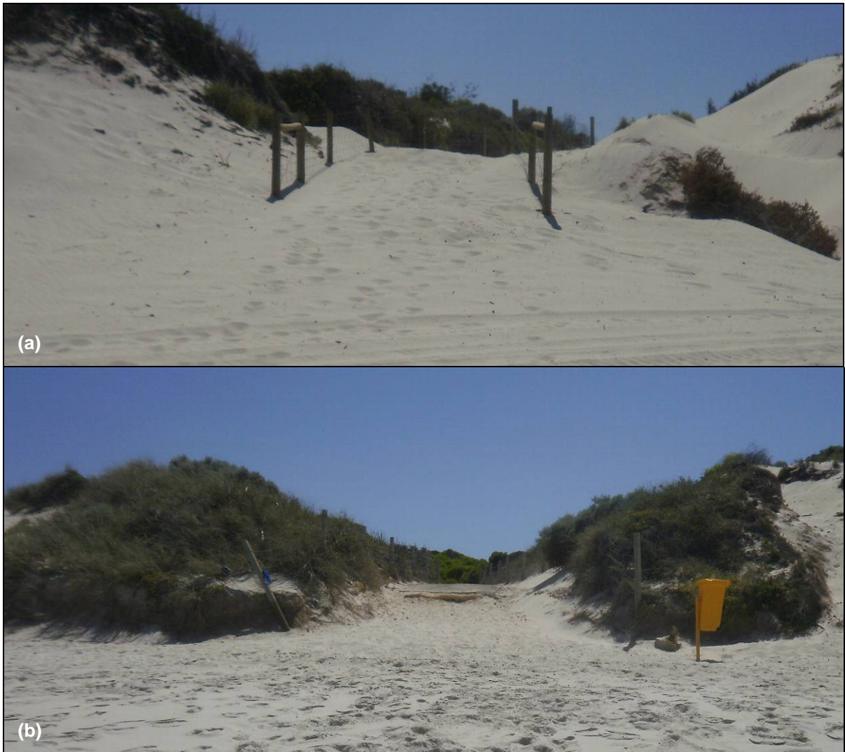
Figure 2.4 – Hillary Cell Access Tracks, (a) Windblown Accretion at the South End & (b) Erosion at the North End (18/1/12)
