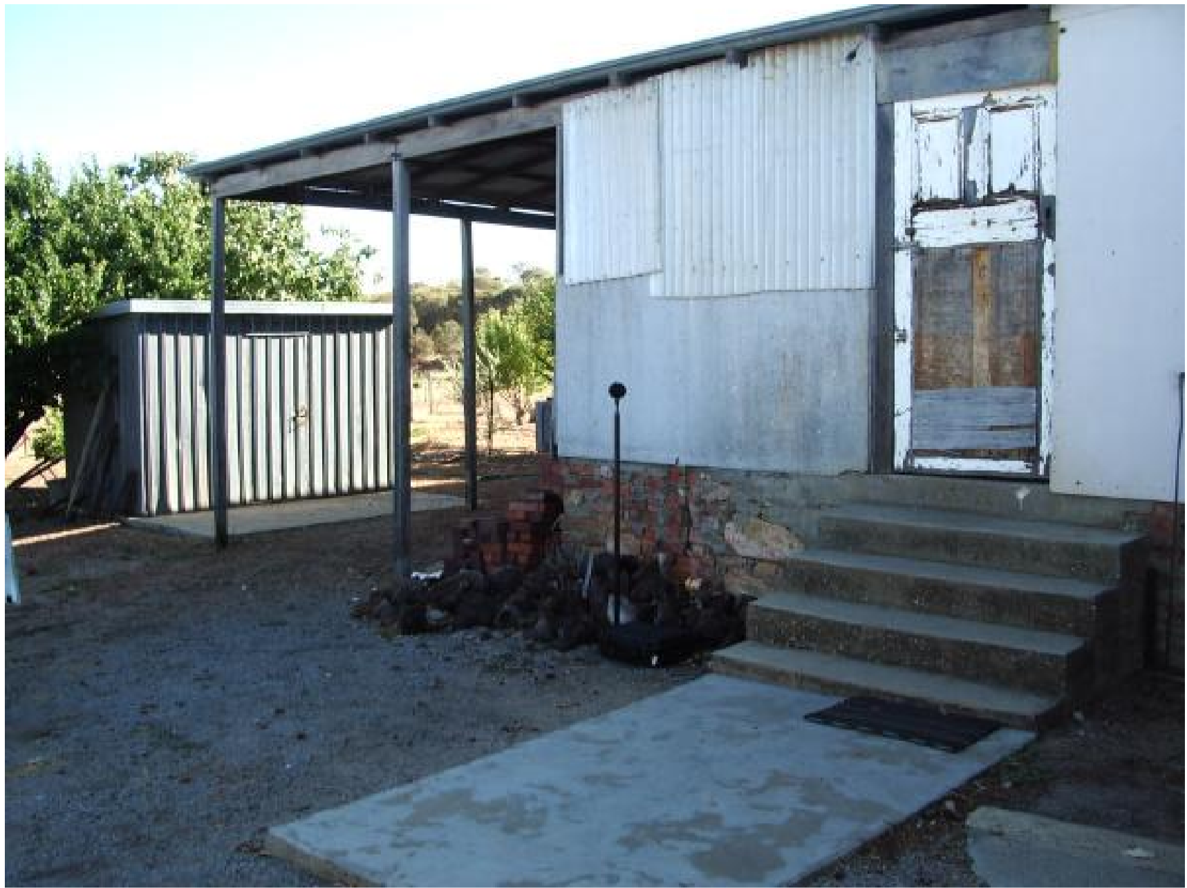
LOCATION 4 – LOT 1 BINDOON – MOORA RD TOWARDS RESIDENCE
