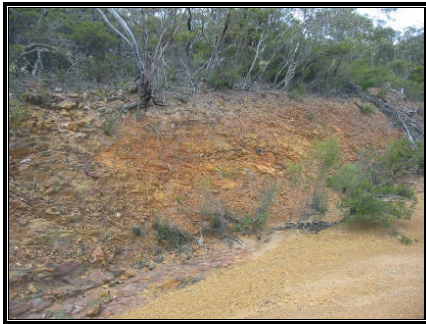
Plate 2 Flag – rocky subsoil at road cutting to north of Flag shaft.
