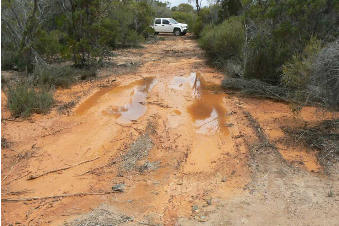
Plate 7 High risk water-gaining site
