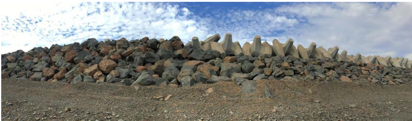
Plate 6: Breakwater wall located at the Port facility
