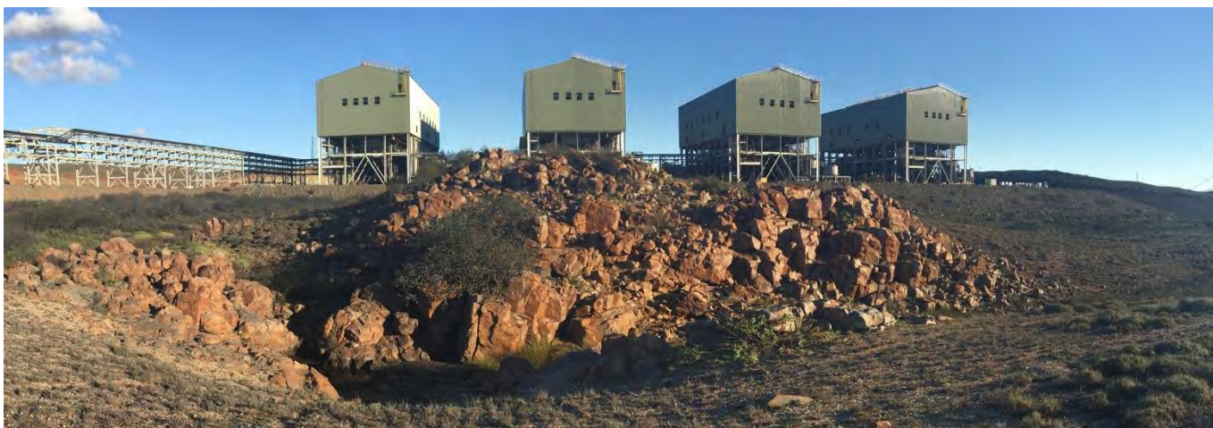
Plate 8: Water seep area located adjacent to the dewatering facility
