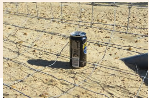
Lapwire installed at the base of the fence can further restrict movement of wildlife such as Echidnas
