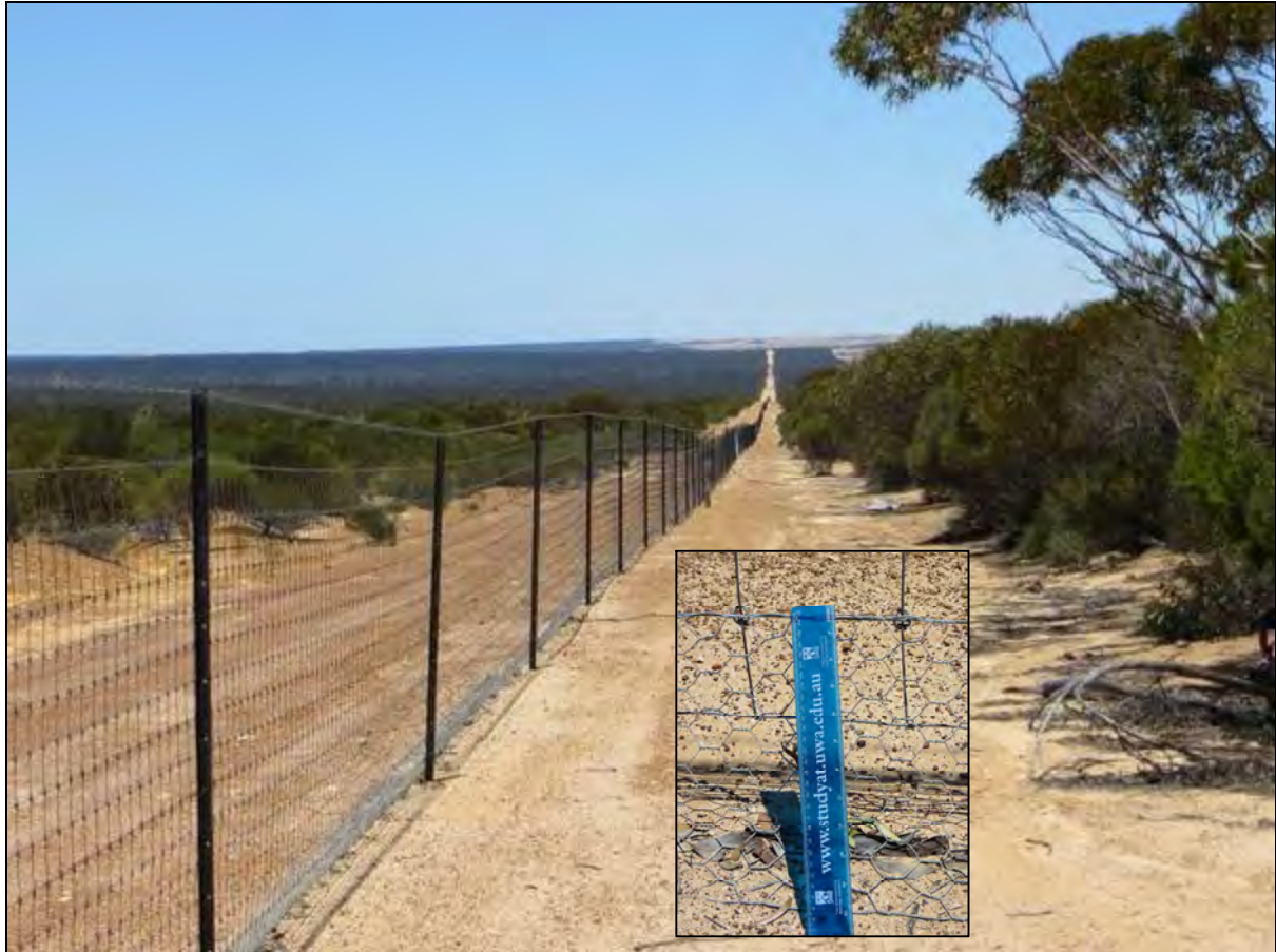
Figure 2: State Barrier Fence east of Hyden. Note the insert shows the lapwire in this location constructed with small aperture 'chicken wire'.
