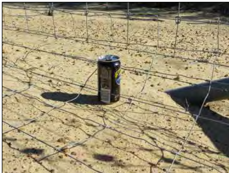
Figure 3: Example of lapwire on the State Barrier Fence without 'chicken wire'
