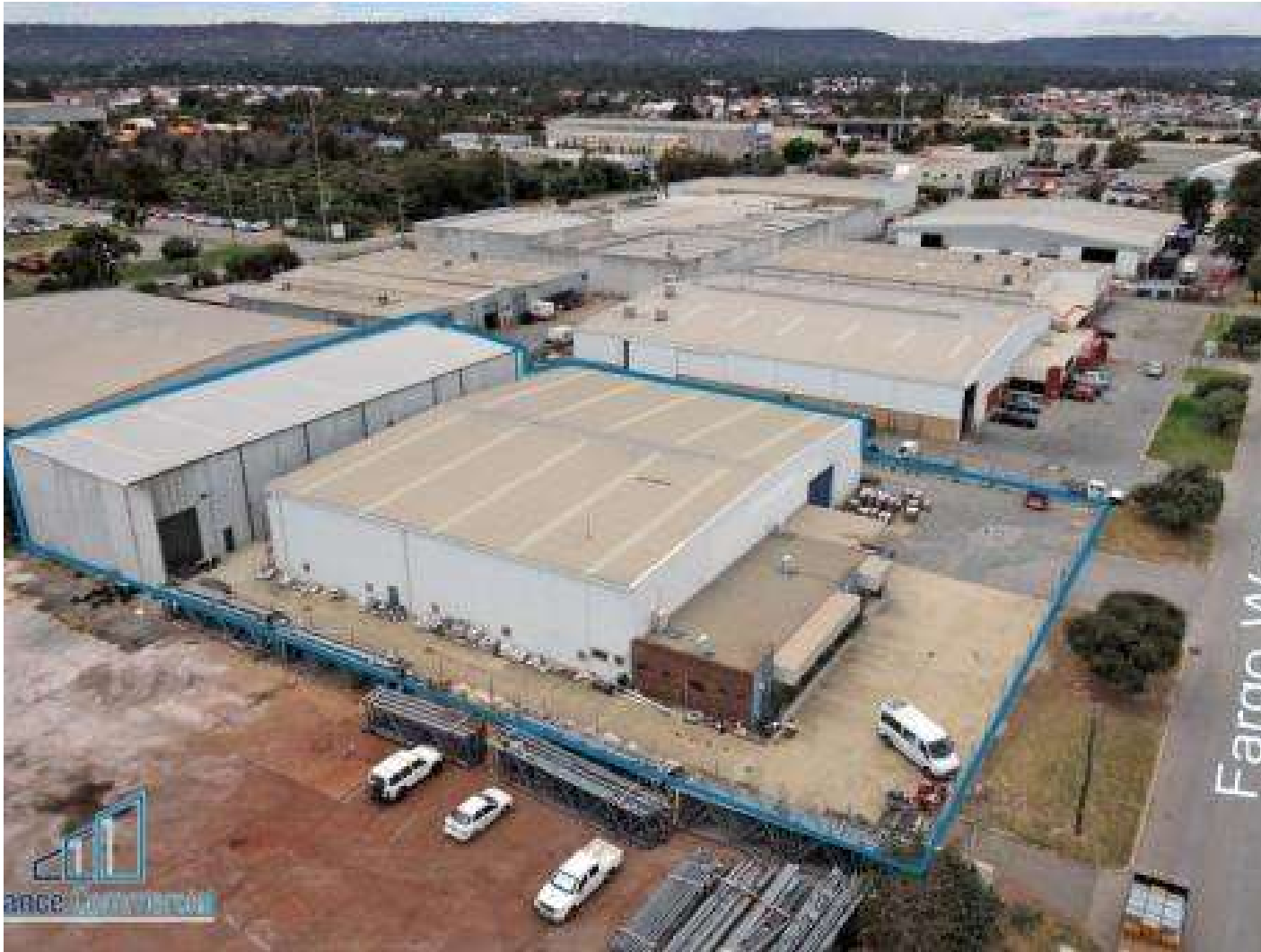
Figure 1: Overview of the proposed site
