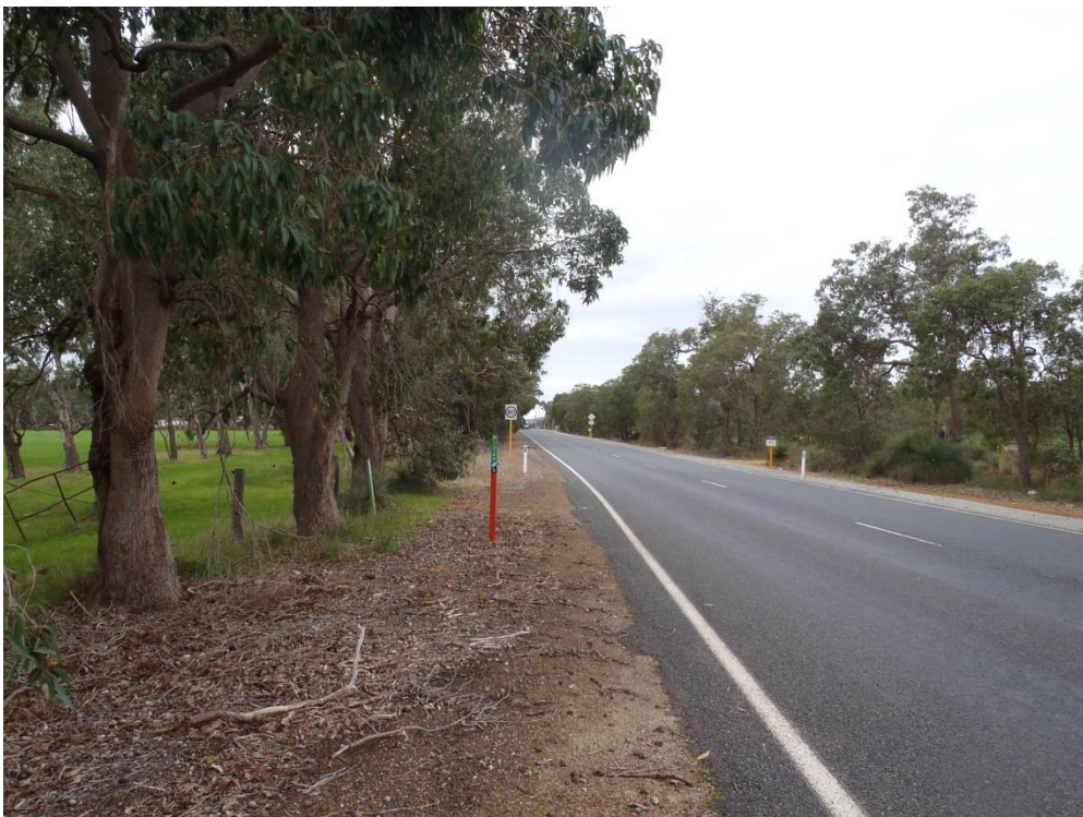
Plate 5: Looking north along Soldiers Road, south of Karbro Road. Pressure main alignment is located directly adjacent to bituminised portion of road, given width in cleared road reserve/road formation this section to be trenched.
