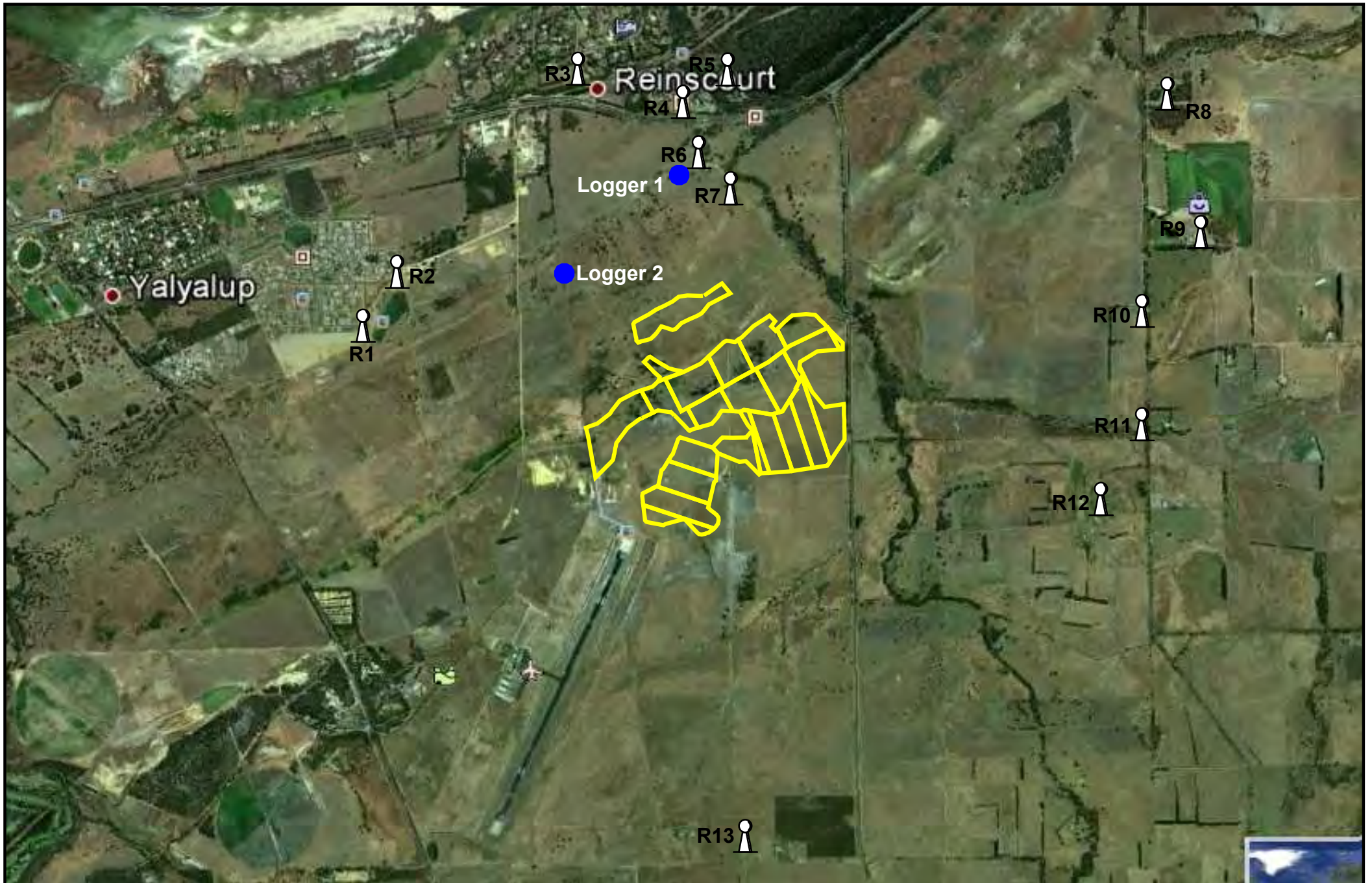
Figure 1: Aerial view of the Wonnerup South Mine site and surrounding area.
