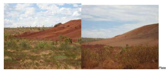
Illustration of a concave slope design (left photo with topsoil applied, right photo without topsoil)
